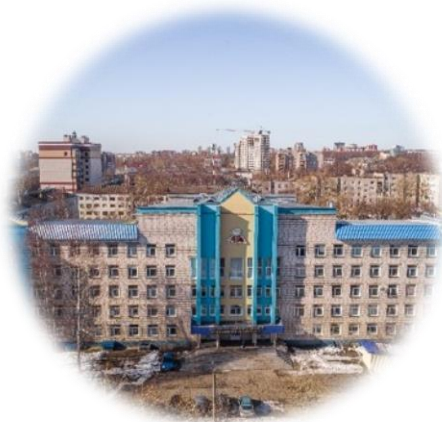
Building 1 137 Karl Marx St
